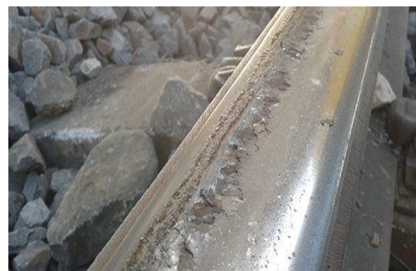
Figure 1: Example of rolling contact fatigue, an indentation in the running surface caused by subsurface fatigue crack [1]
